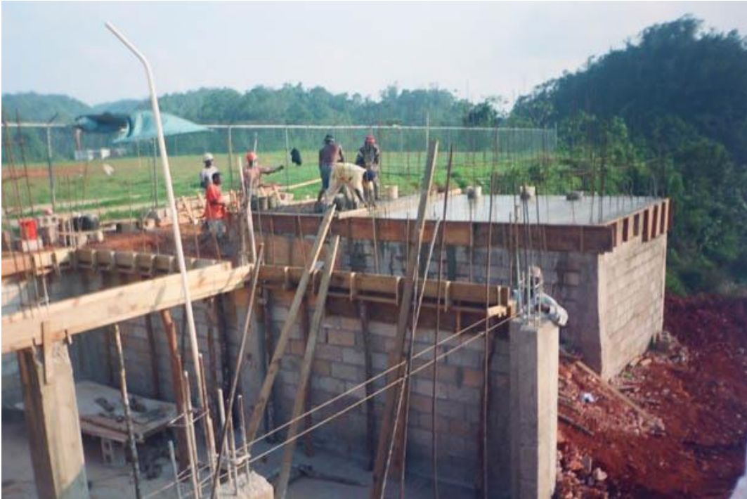
Column & Tie-beams for Classroom Toilet floor being poured
