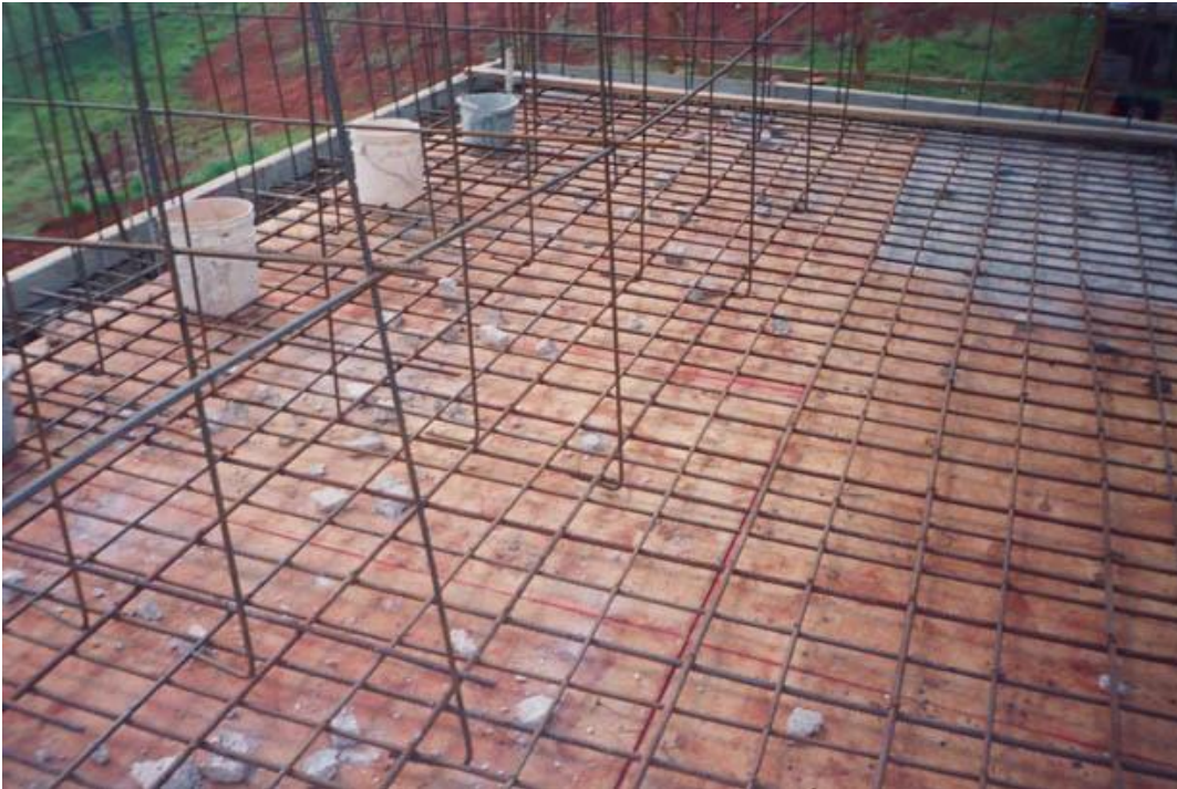
Toilet partition wall framing
