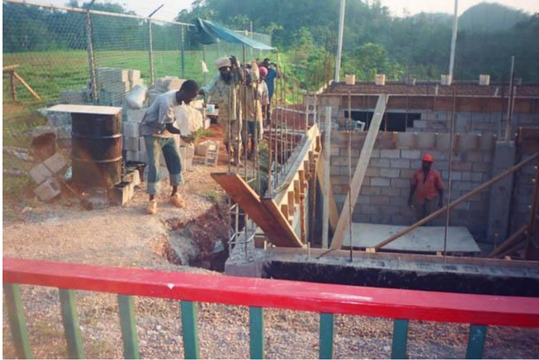
Completing the Storage Basement (with Toilet Building in the background)
