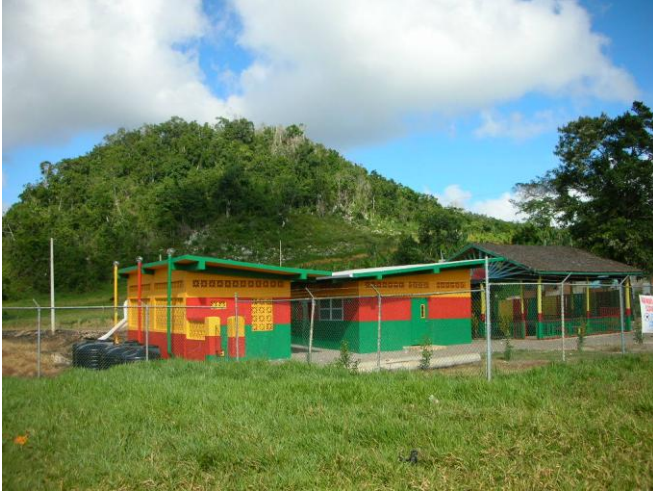
View of new toilet building, new classroom & the outdoor pavilion.
